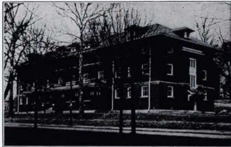
OHIO UNIVERSITY Boyd Hall—A Women's Dormitory
