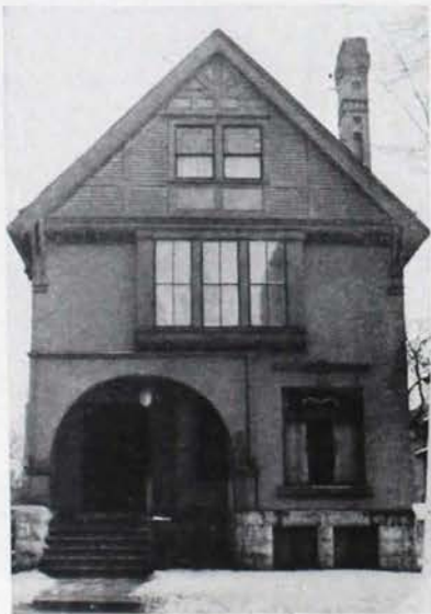
DELTA CHAPTER HOUSE AT MARQUETTE, 604 N. 14th Street, Milwaukee
