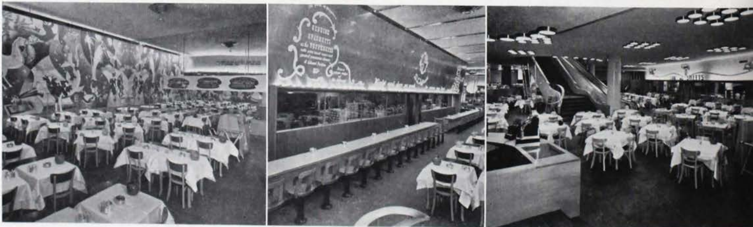
THREE INTERIOR VIEWS OF THE TOFFENETTI RESTAURANT, NEW YORK CITY
