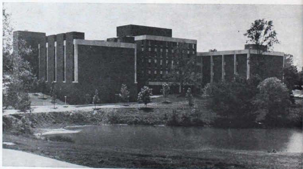
THIS MULTI-PURPOSE complex on the University of Missouri campus at St. Louis houses classrooms, laboratories and faculty offices.
