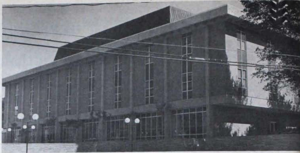
A LONG AWAITED dream of the School of Business and Applied Arts at Sam Houston State College in Huntsville, Texas, is the new building just recently completed.
