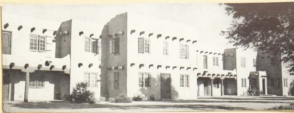
Yatoka Hall, Home of the Business Administration Students
